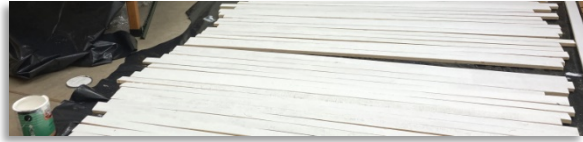
Figure 22. Boards painted white in preparation for masking. Line the boards up side by side for bulk painting. All photos in this series: Lindy Hutchinson.
