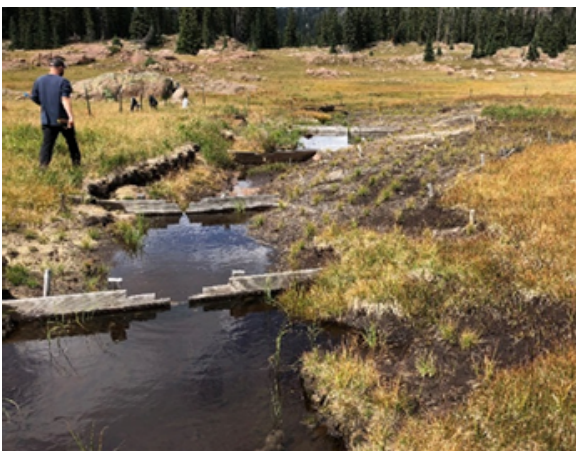
Check dams are slowly restoring groundwater hydrology and allowing vegetation to reestablish (2021)
